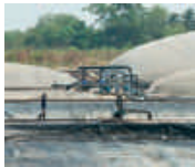
Anaerobic Digestion Plants
